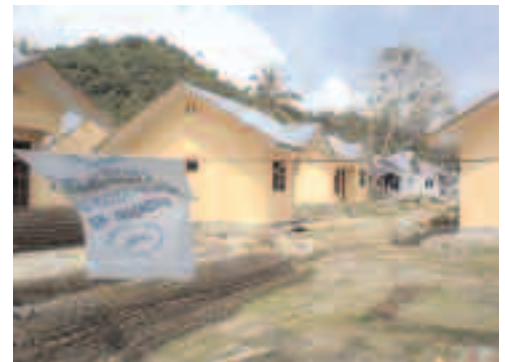
Seibun Ketapang Village under reconstruction by M-USA.
