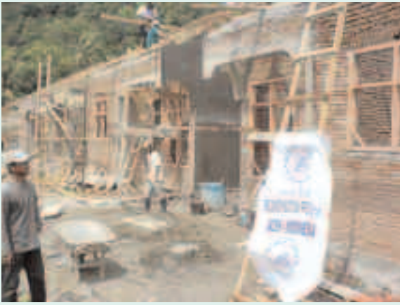
Homes under construction by M-USA in Seibun Ketapang Village..
